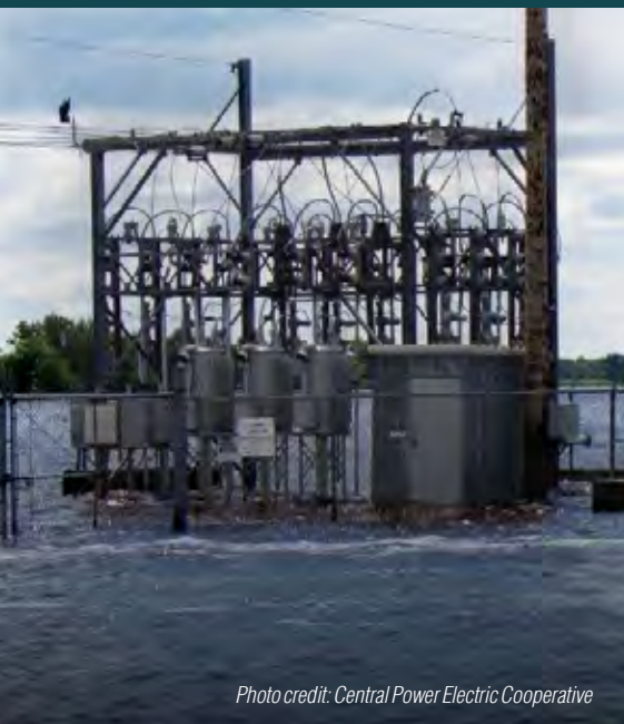
Central Power's Towner distribution substation flooded by the Mouse River.
