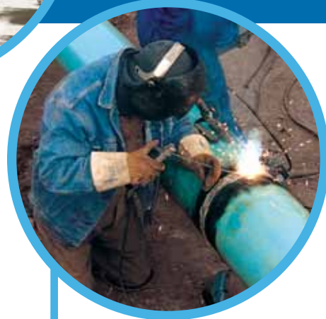
First carbon dioxide enters pipeline from the Synfuels Plant to Canada.
