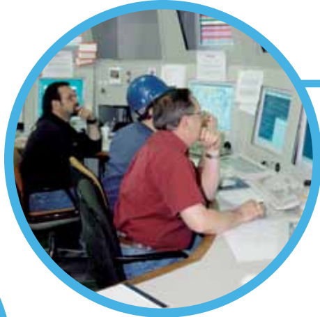
A distributed control system is installed in Unit 2; Unit 1's was installed in 2001.
